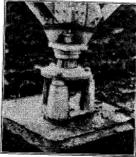
Fig. 13. Close-up view of insulated tower footing.
