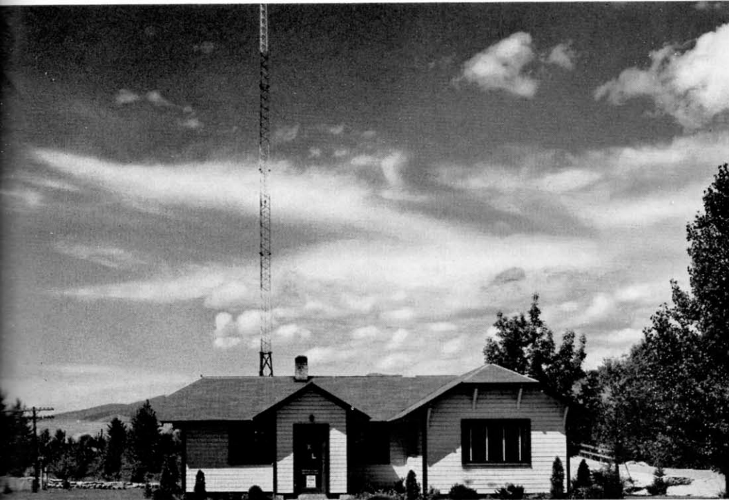
FIG. 1. Shown above is the transmitter building of KXLL which is situated about 200 feet from a river. The antenna tower shown at rear of the building is located at river's edge with half its ground system buried under water.
