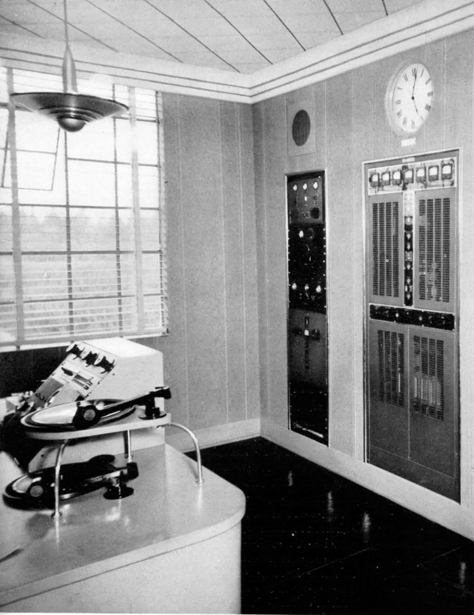
The new Western Electric 310 type transmitter (left) which boosts the station's power from 100 to 250 watts. Dedication programs were heard by New Zealand listeners. The 110A program amplifier is shown at left of transmitter.
