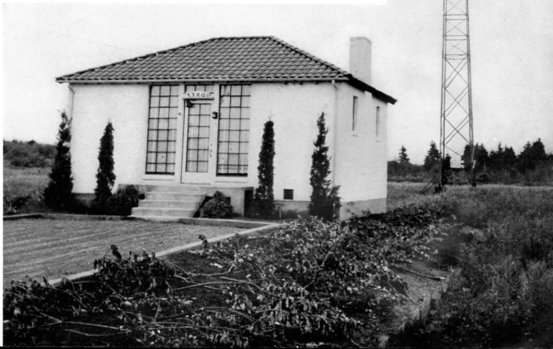
KXRO's modern transmitter building (right) which is constructed of concrete and stucco. The 189 foot Blaw-Knox radiator in background.
