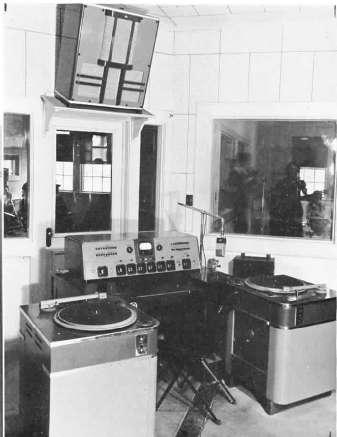
▲ Control room at the Georgia station. Note the similarity to KYUM and WLOK in the arrangement of units.
