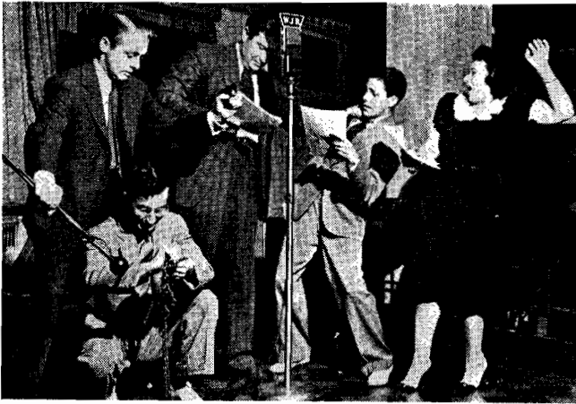
Figure 1 Setup in live-end dead-end studio. (Courtesy Ralph H. Jones Company)
