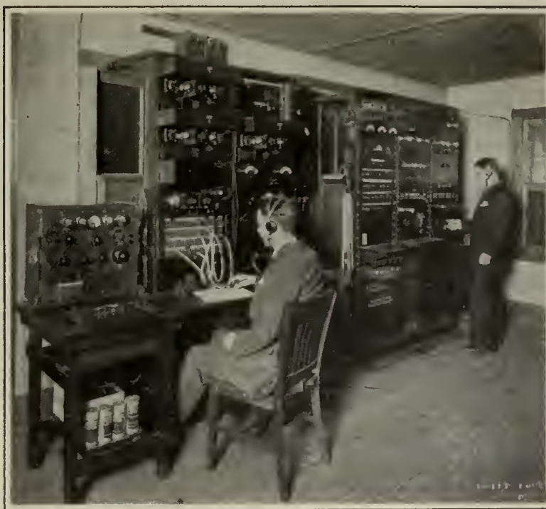
This apparatus is part of that used for the reception of single side-band signals at the Houlton, Maine, station of the American Telephone & Telegraph Co. The operator at the right is adjusting the apparatus used to pick up the signal, and the man at the left is responsible for the wire line to New York
