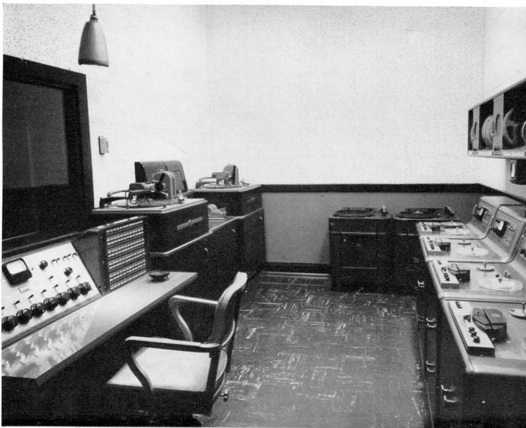
FIG. 48. Interior of the WBT recording room. Control console, at left, faces into Studio C and may be used to control a program originating in this studio independent of master control.
