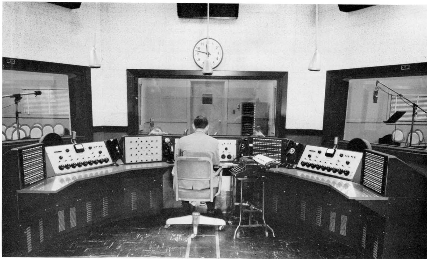
FIG. 45. Master control room of WBT looks into the three radio studios through conveniently placed windows. Master console includes a separate control panel for each studio plus terminal and switching facilities. Studio B (center) is a d.j. studio, equipped with four RCA Type 70-D Turntables and one announcer's control box.
