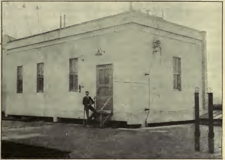
THE TRANSMITTER HOUSE ON TOP OF AEOLIAN HALL
