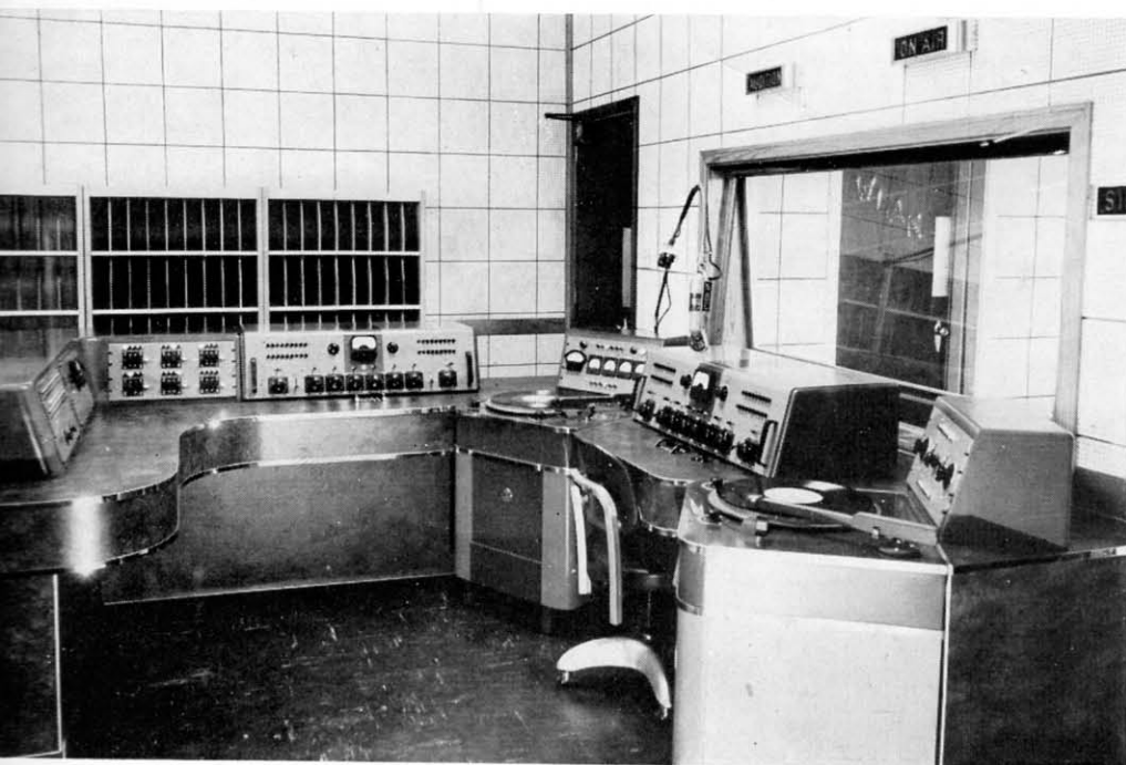
FIG. 1 (above). The WLAKE 1 KW transmitter is visible from window of central control room. Note that monitoring test and audio racks, as well as studio control consoles are all easily reached.
