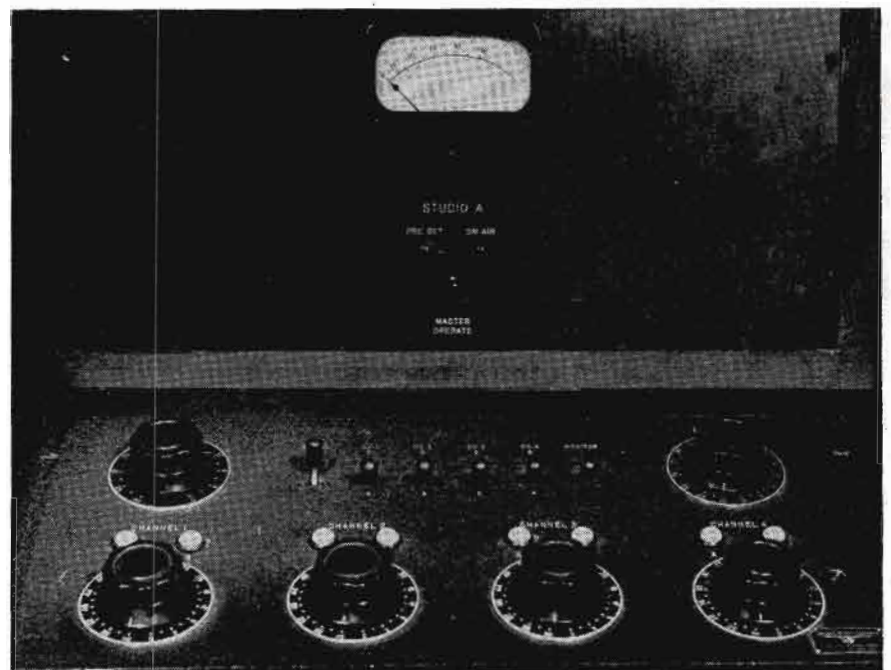
Figure 6 The meter panel of studio A, which is the large auditorium studio. The three master keys are used to switch channels. The key on the left of the mixer panel operates the talk-back relay. Next four keys are for the microphone circuits and the key on the right switches the output of the mixer. When the key is down, the mixer is connected to the amplifier. In the center position, the mixer is off and when up, a trunk is connected to the booster amplifier. This trunk is used to patch to a turntable mixer out for electrical-transcription spots .
