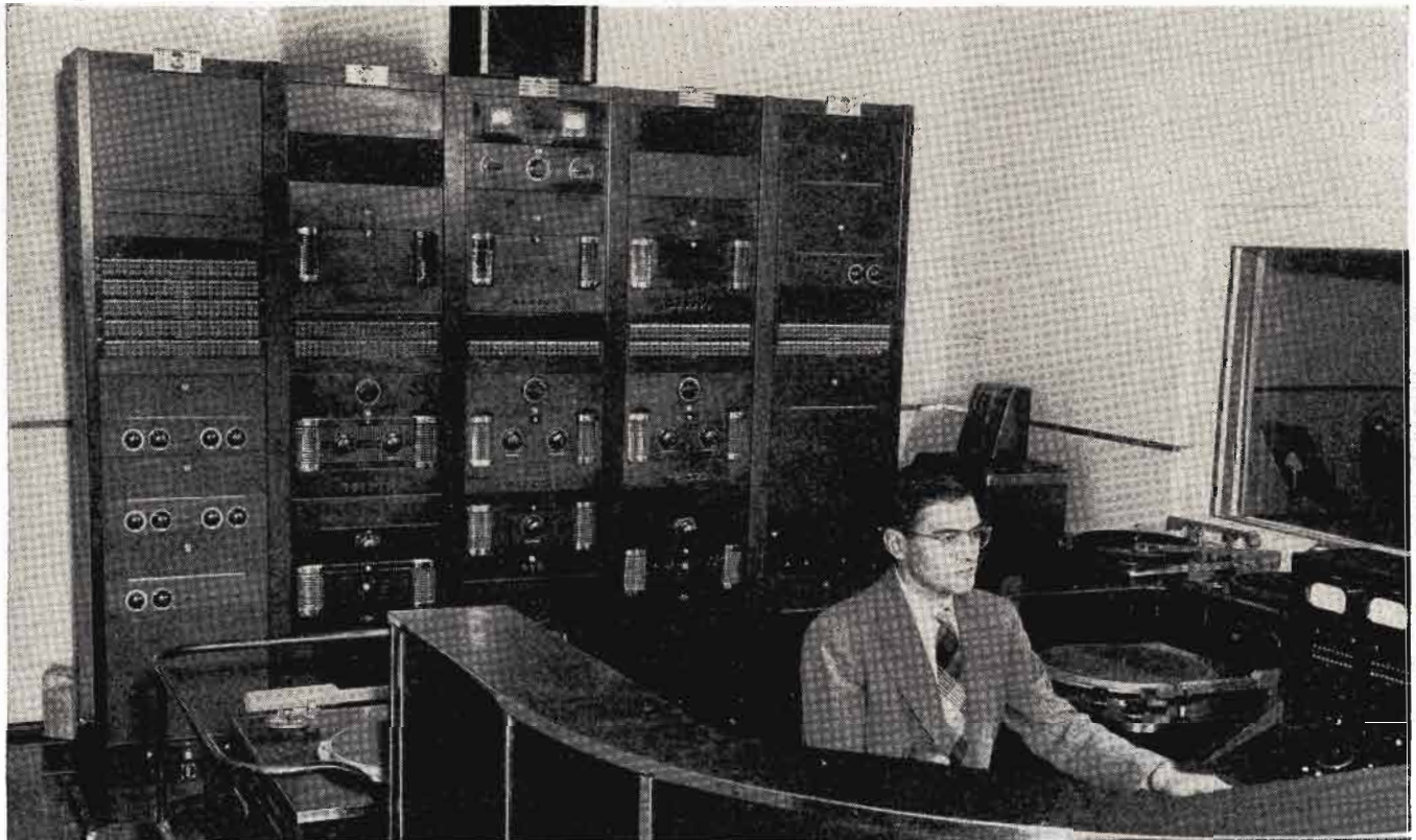
The master control room showing a part of the console, turntables and equipment racks. Rack on left contains the preset switching equipments, while the others contain the equipment for the large auditorium studio (A), medium music studio (B), a-m announcing studio (C), and f-m announcing studio (D).
