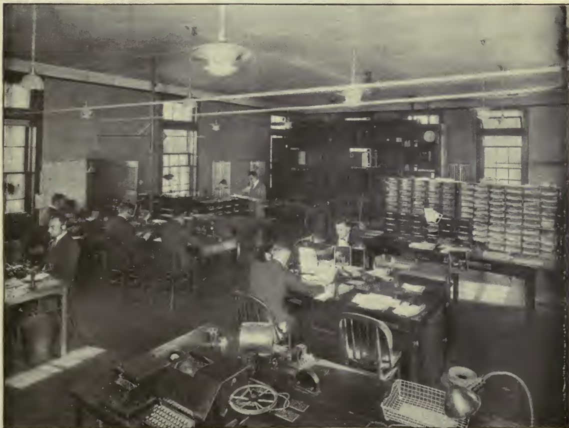
A VIEW OF THE CONTROL STATION AT BROAD STREET, NEW YORK CITY
