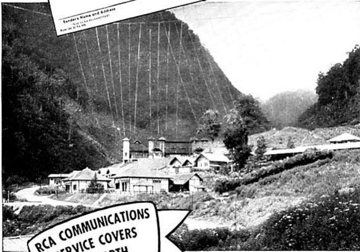
In this scenic tropical setting is located the Malabar transmitting station of the Netherlands East Indies Telegraph Administration. The aerial has been strung from one mountain top to another.
