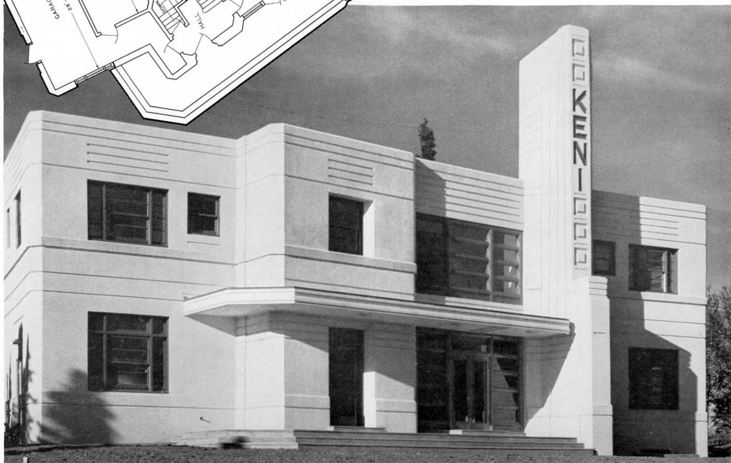
FIG. 1. The modernistic KENI transmitter building is constructed of reinforced concrete. Inset at upper left shows layout of garage, transmitter and bachelor apartment facilities on the main floor of the building.
