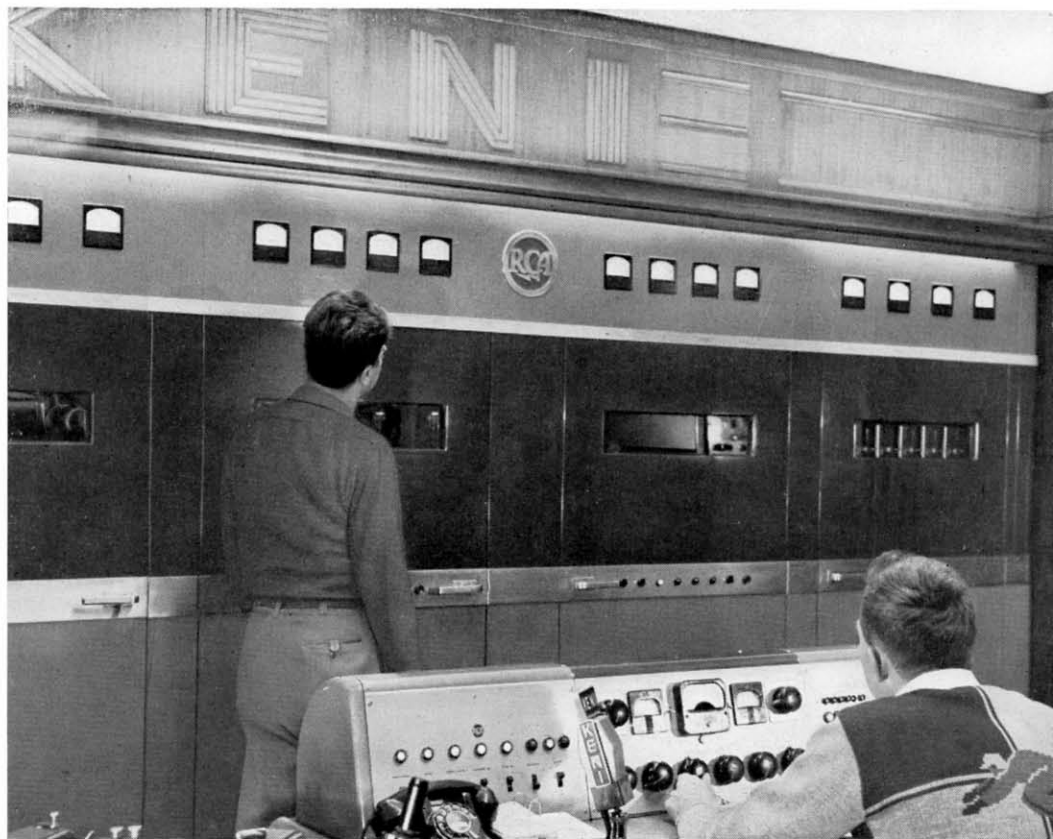
FIG. 3. Engineer Ray Walker checks the meters on the KENI transmitter, RCA Type BTA-5F. Chief Engineer Jack Walden is at transmitter console controls.
