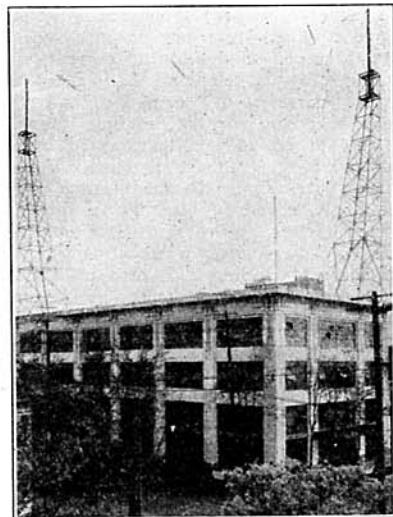
Aerial at KFI Supported by Roof. 96 ft. Steel Towers and 25 ft. Masts so as to be 175 ft. Above Ground.
