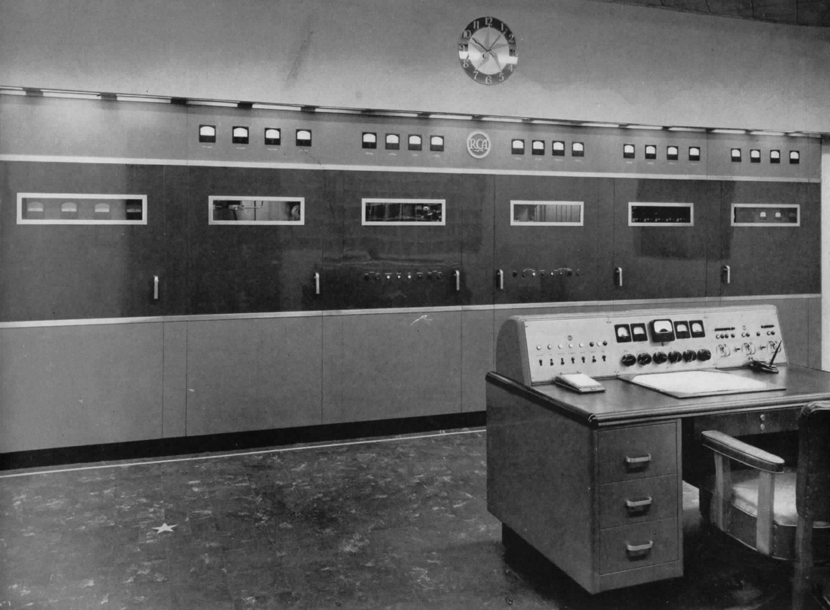
KMPC TRANSMITTER ROOM —The 10-E transmitter, the phasing equipment for the three-tower antenna array, and the speech input and monitoring equipment are all mounted behind the single "unified-front" type enclosure shown above. The operator's console and a monitoring speaker mounted in the ceiling are the only other items of equipment in the transmitter room. The extra panel units which make this ultra-streamlined installation possible are optional accessories with the 5-E and 10-E transmitters.
