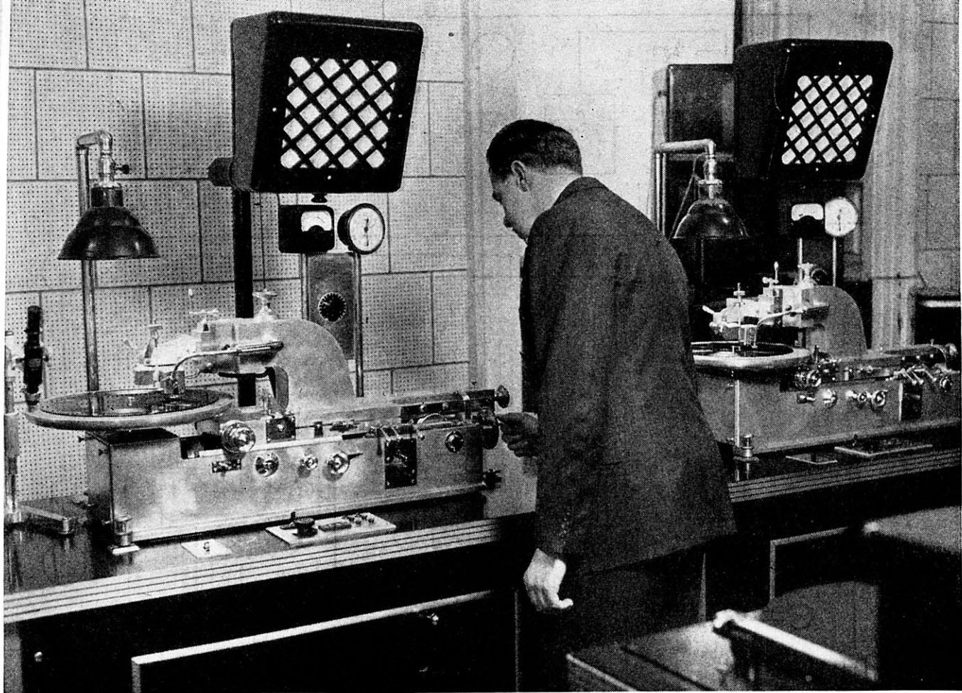
Adjusting the feed mechanism on one of the Scully recorders. Controls in foreground are for the automatic relay system, head controls and a variable control for adjusting the program monitor output.
