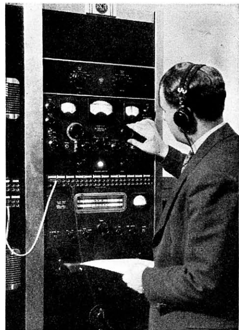
John Langenegger, Chief Engineer of the Library of Congress Recording Laboratory, shown tuning in on the Hallicrafters SX-28 receiver. The high-fidelity AM-FM tuner is shown mounted below the SX-28.
