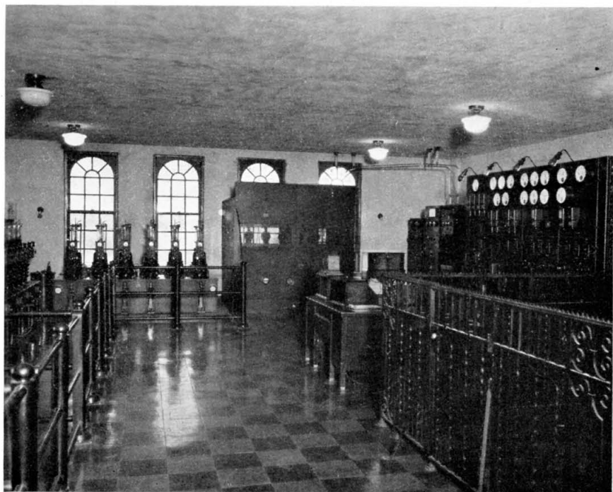
FIGURE 2—NEW RCA RECTIFIER, CENTER PANEL
