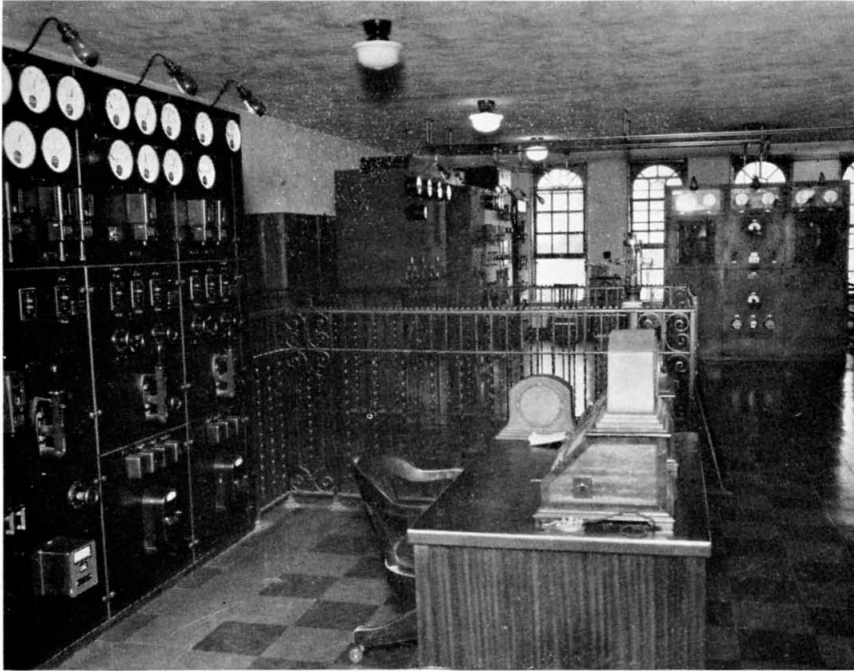
FIGURE 1—RCA 50 K. W. AMPLIFIER, FAR END OF ROOM. 5 K. W. TRANSMITTER AT LEFT END
