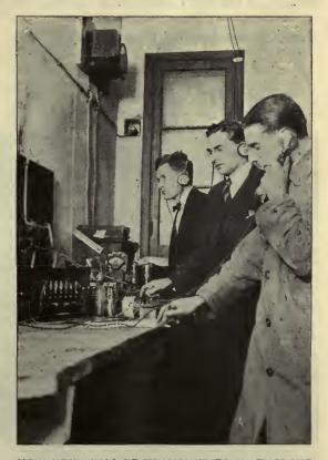
HOW KDKA WAS RE-TRANSMITTED IN ENGLAND The receiving set had six stages of tuned radio-frequency amplification, detector and two stages of audio-frequency amplification. This special station is installed at Biggin Hill, near Manchester. In the photograph are, *left to right* Mr. Honri, of the British Broadcasting Company, Mr. Webb, of *Popular Wireless*, and Captain West, Assistant Chief Engineer
