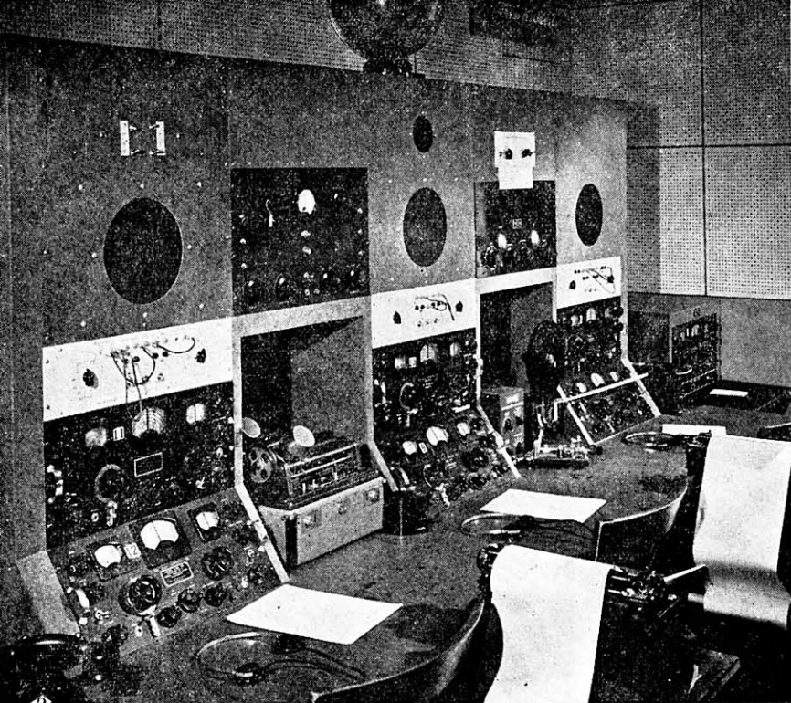
A "ham's paradise." Any type of signal may be recorded in the Intercept Room on tape, wax cylinders, or paper discs for observation and reference.
