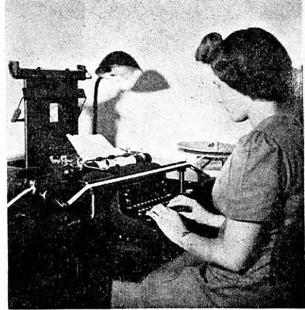
Transcribing copy from Boehme tape. Operator controls speed by foot.
