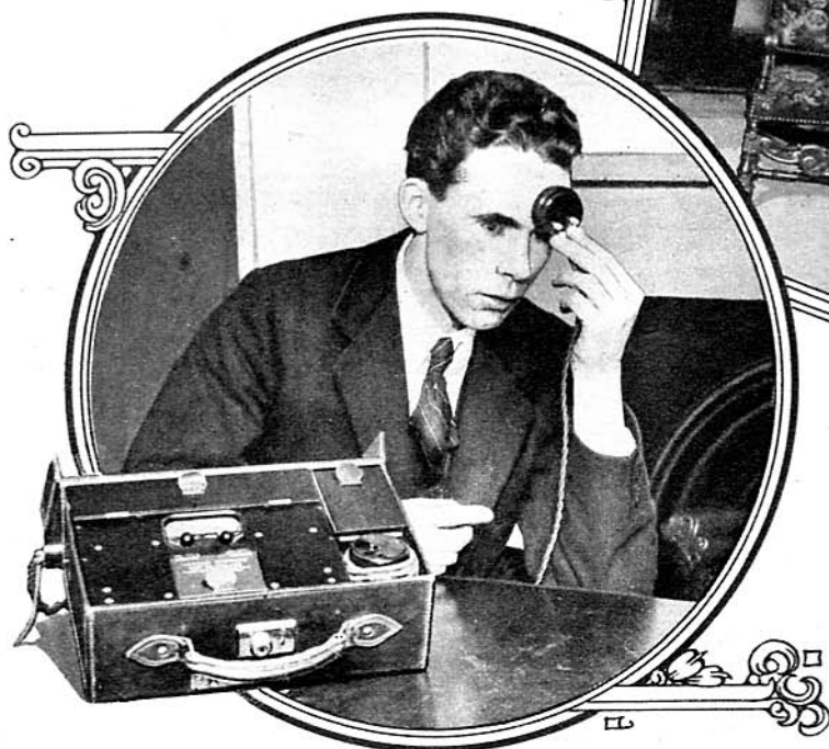
RADIO FOR THE DEAF has been made possible by this new device shown at the recent Medical Exhibition at Westminster, in England. The set is of ordinary type, employing two vacuum tubes. The contact device, which takes the place of the usual headphones, when placed against the elbow, knee or forehead, faithfully imparts the vibrations to the bones of the listener, which in turn affect the auditory nerves. It has been stated that a lady visitor to the Exhibition, who had not heard for 40 years, was able to hear music through the medium of this instrument.
