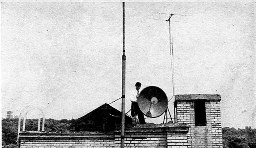
Engineer Tom Humphrey makes an adjustment on the studio-transmitter radio link microwave dish antenna which beams programs from atop the Ithaca Savings Bank Bldg. to Connecticut Hill, whence they are channeled to six other stations in net.
