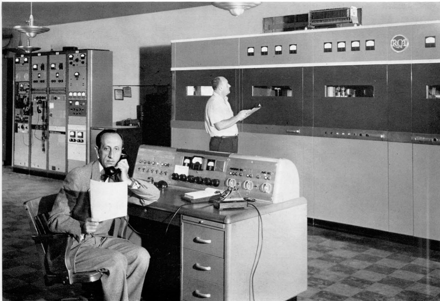
FIG. 11. Harry Dennis, Chief Engineer, at control desk in transmitter room. In background is John Geczi, Transmitter Engineer, at RCA Type BTA-5F 5-KW Transmitter. To the left are the audio racks. (Not seen at extreme left, is RCA Type BTF-10B 10KW FM Transmitter.)
