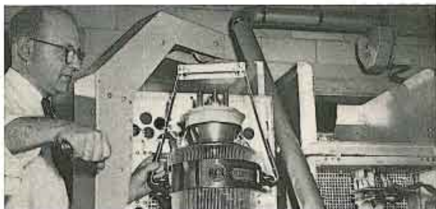
A. B. Van Alstyne, WTMJ transmitter supervisor, using a tube hoist to remove one of the 6592 power amplifier tubes.
