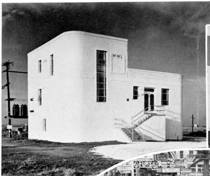
Above: Transmitter House—WWL.
