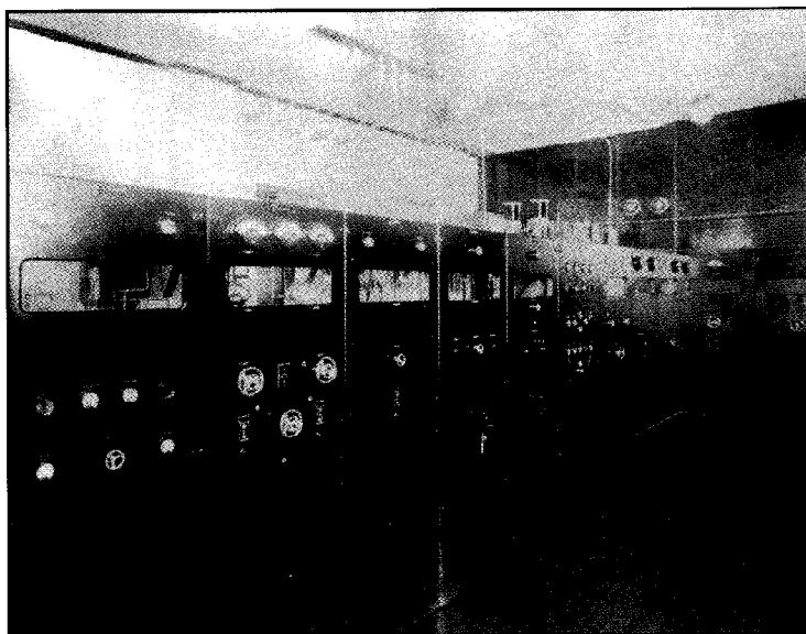
Figure 5. Control panels for the 180-kw station. The modulator tubes in Figure 3 are behind the third and fourth panels from the left, and the power amplifier tubes are behind the eighth and ninth panels. The tank circuit in Figure 4 is on the other side of the wall at the far right in the figure. The plate leads connect to the tank circuit through the feed-through insulators that are visible on the wall.
