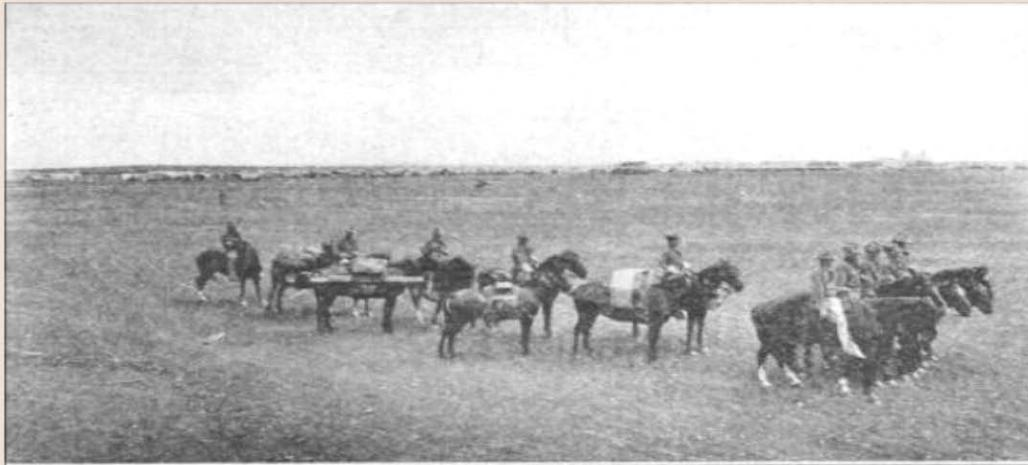
Fig. 107.—Company D Signal Corps at San Antonio, Texas, 1911, showing pack sets and telescoping pole carried by pack mules.
