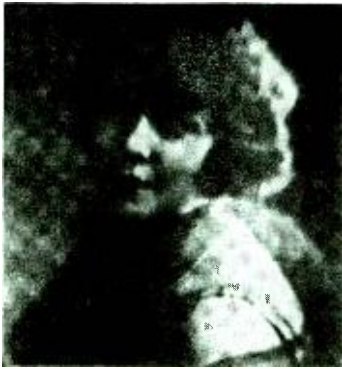
Two photographs after they had been transmitted a distance of eighteen miles by the Jenkins television apparatus.
