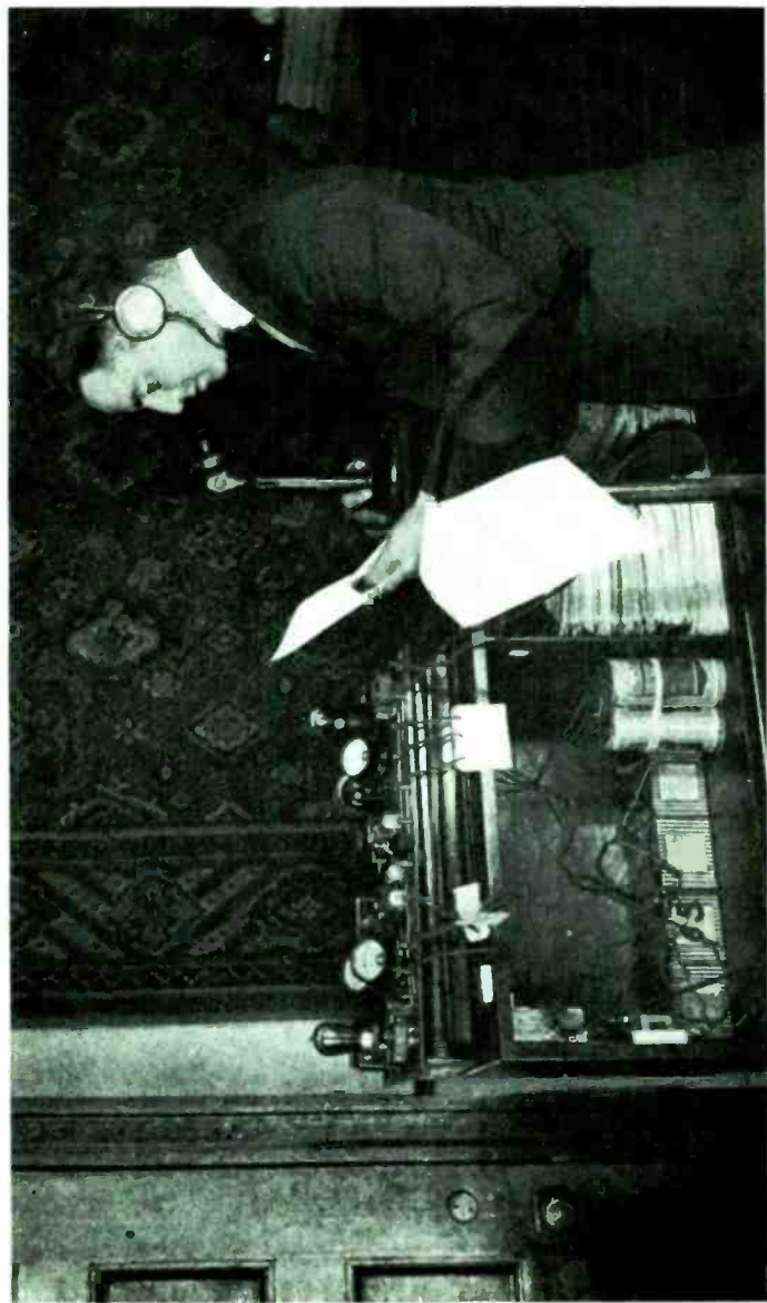
WGY's dramatic director, Mr. Smith, at the telephone. At the left are two stages of amplification, one stage to amplify the voices from the studio for reception on the phones and the second stage to amplify the voice of the director which reaches the players through the loud-speaker.
