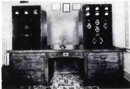
THE OLD POLICE TRANSMITTER EQUIPMENT OF KGPE, WHICH IS NOW BEING RETAINED AS AN AUXILIARY
