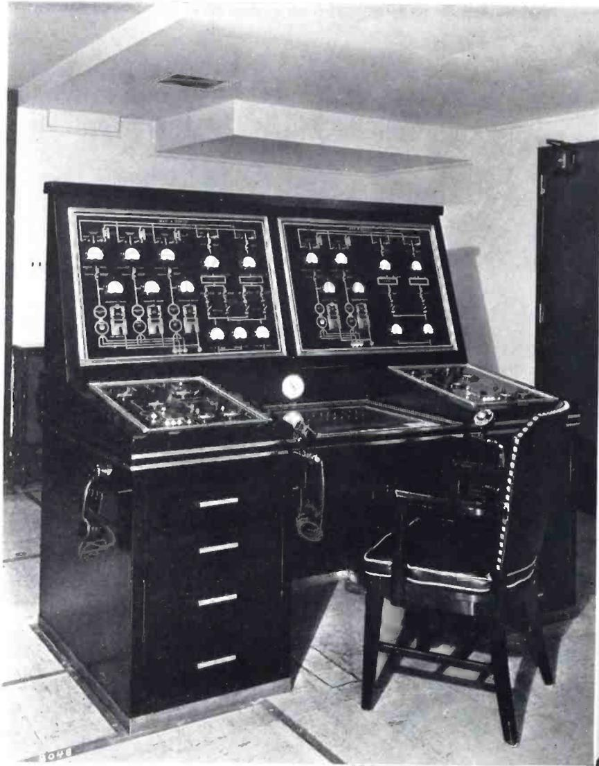
(ABOVE) POWER CONTROL DESK SHOWING POWER CIRCUITS IN MINIATURE, TOGETHER WITH INDICATING METERS AND LIGHTS. THIS DESK IS THE REMOTE CONTROL POINT FOR ALL OF THE POWER EQUIPMENT
