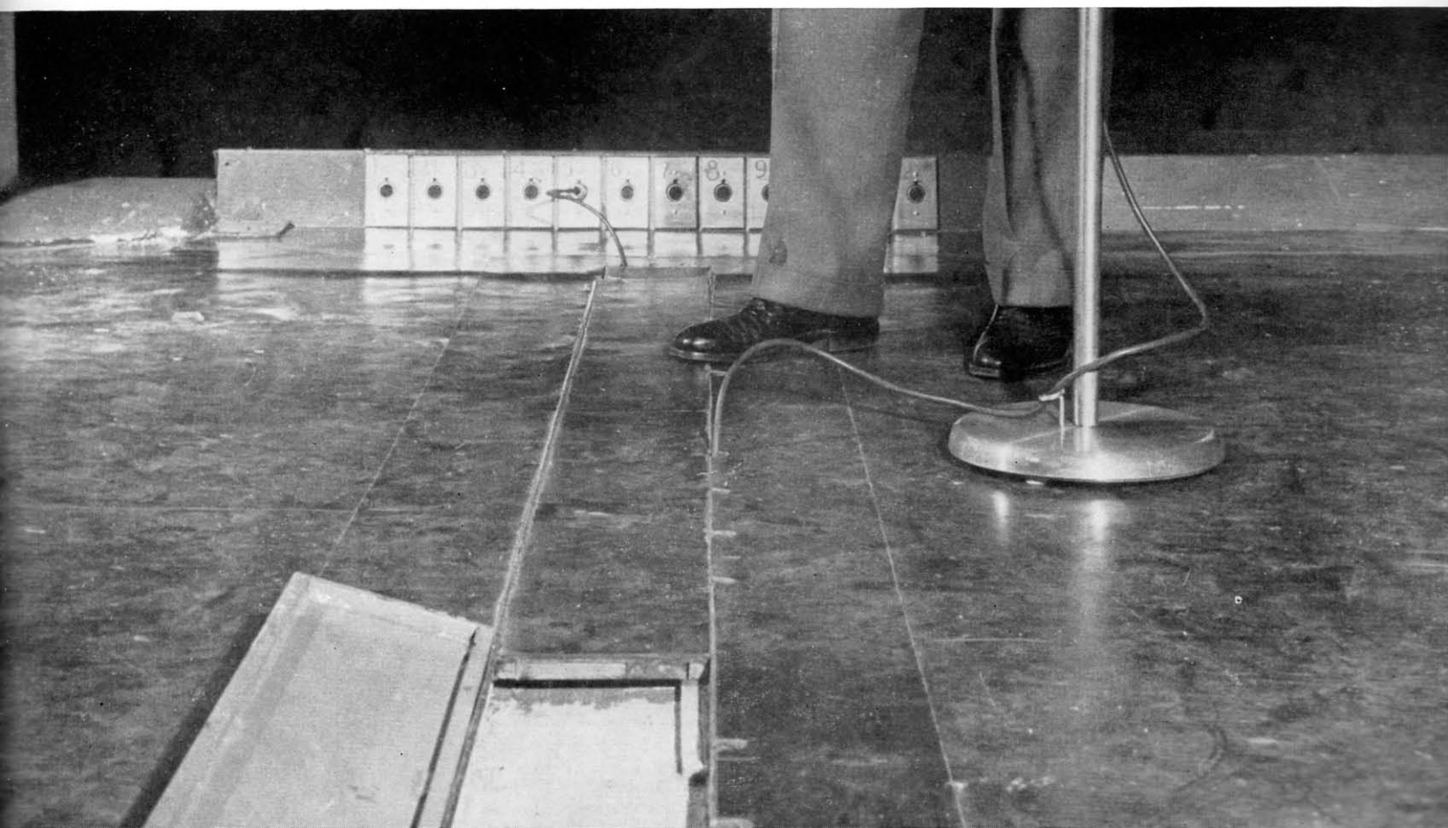
FIG. 9. Twelve microphone receptacles are mounted across the front of the stage. Note hinged floor boards for mike cords.
