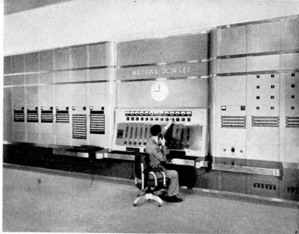
View of the Master Control above shows the operator adjusting signal level on an outgoing line, with VU meter above gain control as guide.
