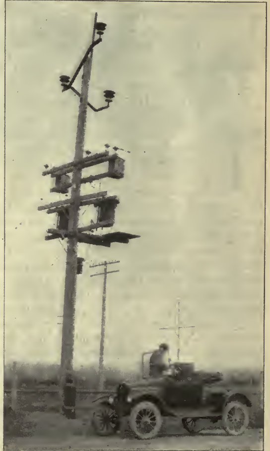
TESTING A TRANSFORMER
