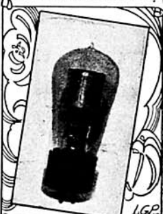
Helium Rectifier; 250 ma. Output for "A" Eliminators. About 1925-6.
