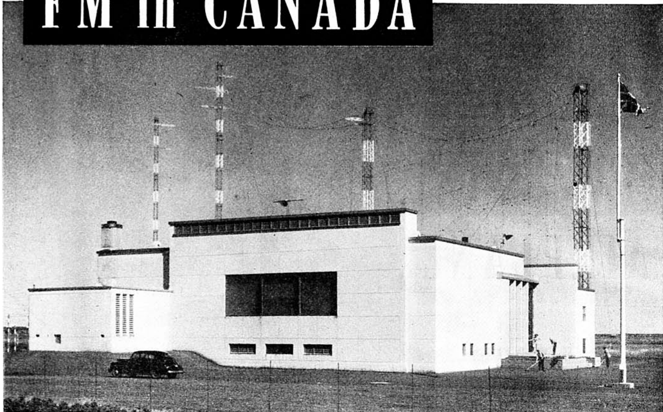
Transmitter building located at the new CBC International Short-wave Service at Sackville, N. B. This building also houses the 50-kw. transmitter for CBA, which is Canada's regional station for the Maritimes. The CBA antenna is to the left of the building shown in the photograph, but the tower itself cannot be seen. The antenna behind the building is used exclusively for the Short-wave Service.
