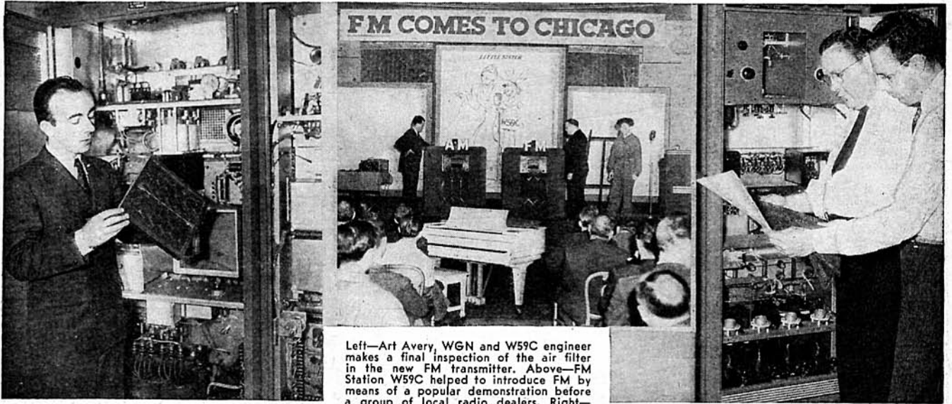
Left—Art Avery, WGN and W59C engineer makes a final inspection of the air filter in the new FM transmitter. Above—FM Station W59C helped to introduce FM by means of a popular demonstration before a group of local radio dealers. Right—Carl J. Meyers, Chief Engineer of WGN and W59C (left) and his Assistant, Clyde White, during installation of FM transmitter.
