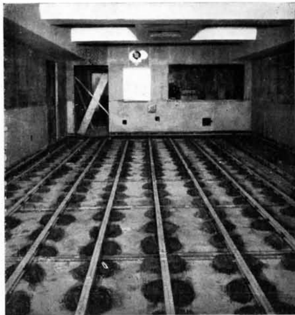
Figure 4. Anchor legs fastened to floor by cement blocks.
