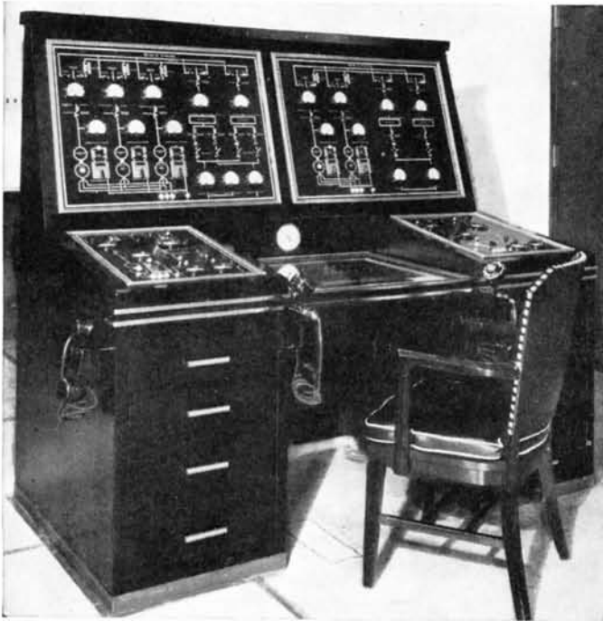
Figure 32. The power control desk showing the miniature supervisory equipment on the panels.
