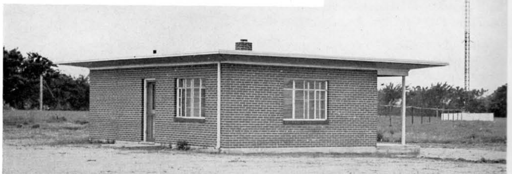
FIG. 3. KAKE's transmitter plant is a one-floor, brick-constructed building occupying a space of only 24' x 29' (approximately). Antenna tower is visible at right.
