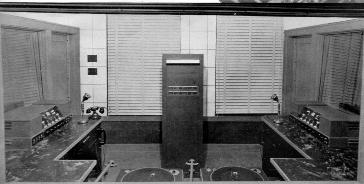
Below: Twin 23A speech input equipments afford maximum flexibility of control. For remote programs KSAL uses the 22A.
