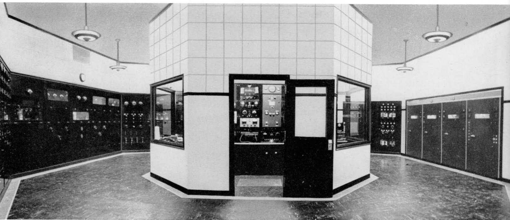
FIG. 1. Interior of transmitter building at KSTP looking toward the rear of the octagonally shaped room. At the far right, the four cubicles of the BTA-50G 50 KW AM Transmitter can be seen. Just to the left of the BTA-50G is a composite 1-kw stand-by transmitter housed in two cabinets. The control room at the center of the main transmitter room contains the transmitter test and measuring equipment as well as facilities for programming of records and station breaks. At the left of the control room, a portion of the old composite 50-kw AM transmitter can be seen. This composite 50-kw unit takes up approximately one-half of the wall space of the transmitter room. In contrast to this, the new BTA-50G occupies less than 15 feet of wall space—an area formerly occupied by a 10-kw FM transmitter.
