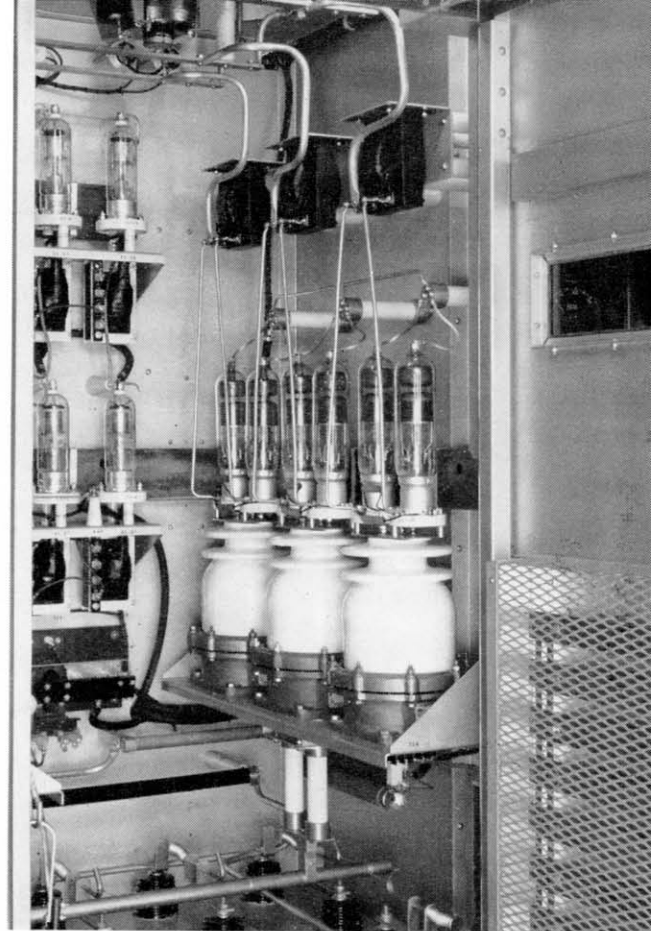
FIG. 3. Rectifier cabinet, front view, showing high voltage rectifier filament transformers and the low voltage 8008 supply. To facilitate remote control, the rectifier cabinet is air conditioned. The unit mounted on the front door is a thermostatically controlled heater. This heater, in conjunction with an exhaust fan, keeps the internal temperature of the cabinet within the operating limits of the mercury vapor rectifier tubes when the transmitter is in operation.
