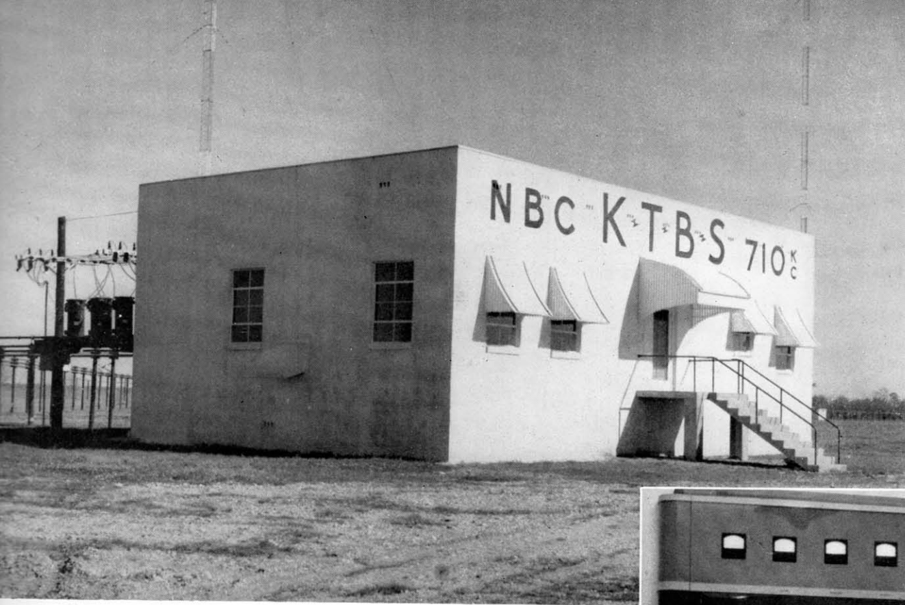
FIG. 1 (above). KTBS' new transmitter building is located 14 miles northwest of Shreveport. Floor of the fireproof building is five feet above ground level so that equipment is safely above possible flood waters.
