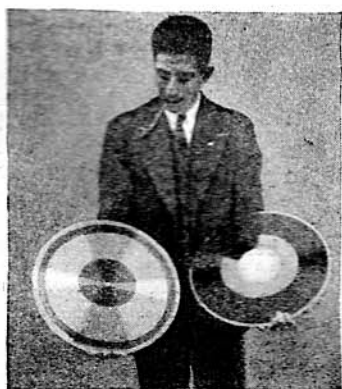
At the left are shown the bright metal stamper which stamps the records and a finished record ready for rebroadcasting purposes
