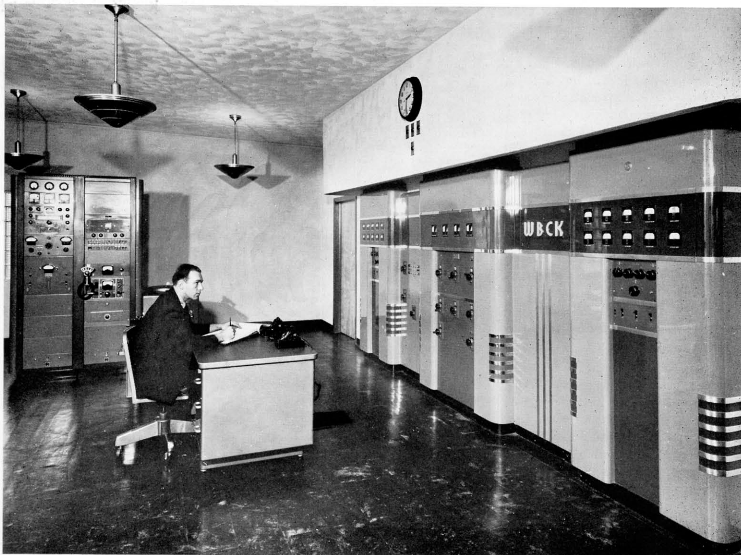
FIG. 1. (below). WBCK's 1 KW transmitter room view showing how phasing equipment is located between the 250-watt exciter and 1 KW amplifier cabinets. Chief Engineer, A. J. Geranis is at transmitter control desk. At far left are test and audio input racks.
