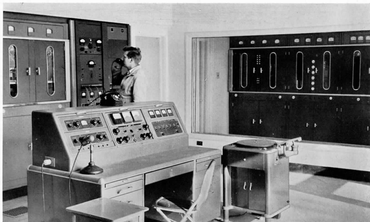
Control room in new dual AM-FM transmitter building for WDNC and WDNC-FM. Console for control of both transmitters in foreground, 5 kw AM transmitter in right rear, and audio and phasing equipment at left across the back of room. The 10 kw FM transmitter faces into room from side opposite the AM equipment.
