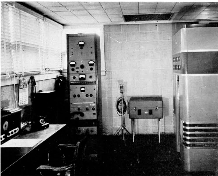
FIG. 3. This photograph of the interior of the WHHM transmitter building shows the operator's desk, the audio and monitor rack, a utility turntable, and the 250-watt RCA transmitter.
