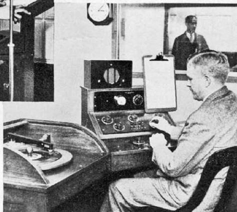
At right, a turntable and control panel for reproducing specially recorded music carried to subscribers by wires
