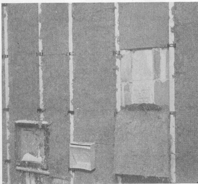
Fig. 7—View of soundproofing on wall (close-up).
