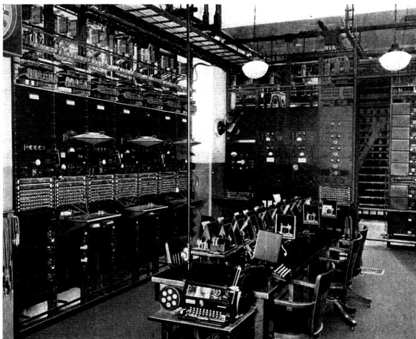
Fig. 5—Portion of Program Apparatus Layout in New York Long Distance Telephone Office as of January 15, 1929.
