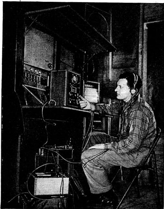
Signal Corps Photo Part of the supersensitive receiver and test equipment used for the measurements.
